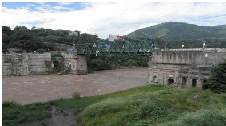
Fig. 5 View of Ranbir Singh Baradar (present condition)
